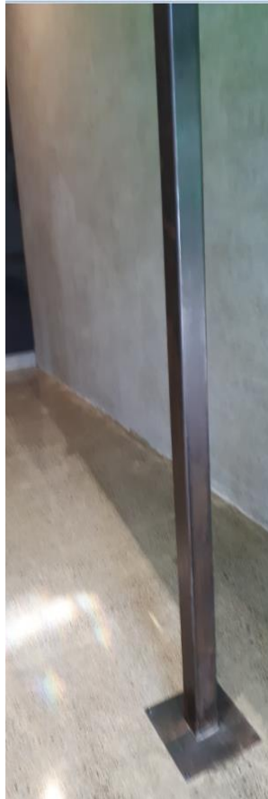
Photo 2 – Ground Floor Metal Pole Under Stairs
